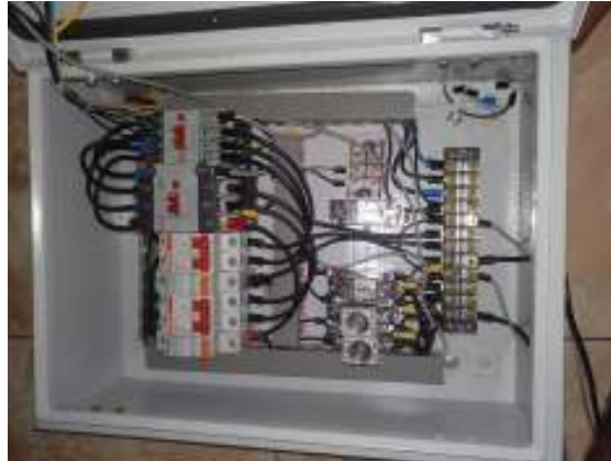
Gambar 2. Rangkaian Multiple Changeover Switch
