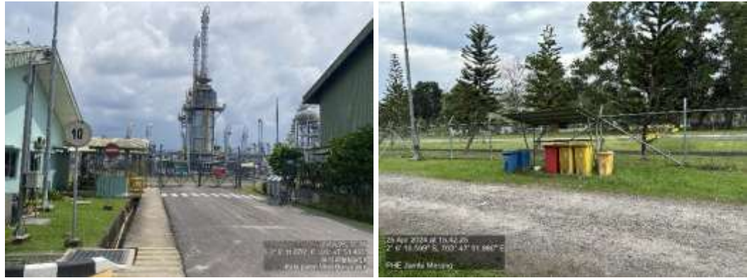
Gambar 3. 8. Area Maintenance Office Work Shop dan CW 7
