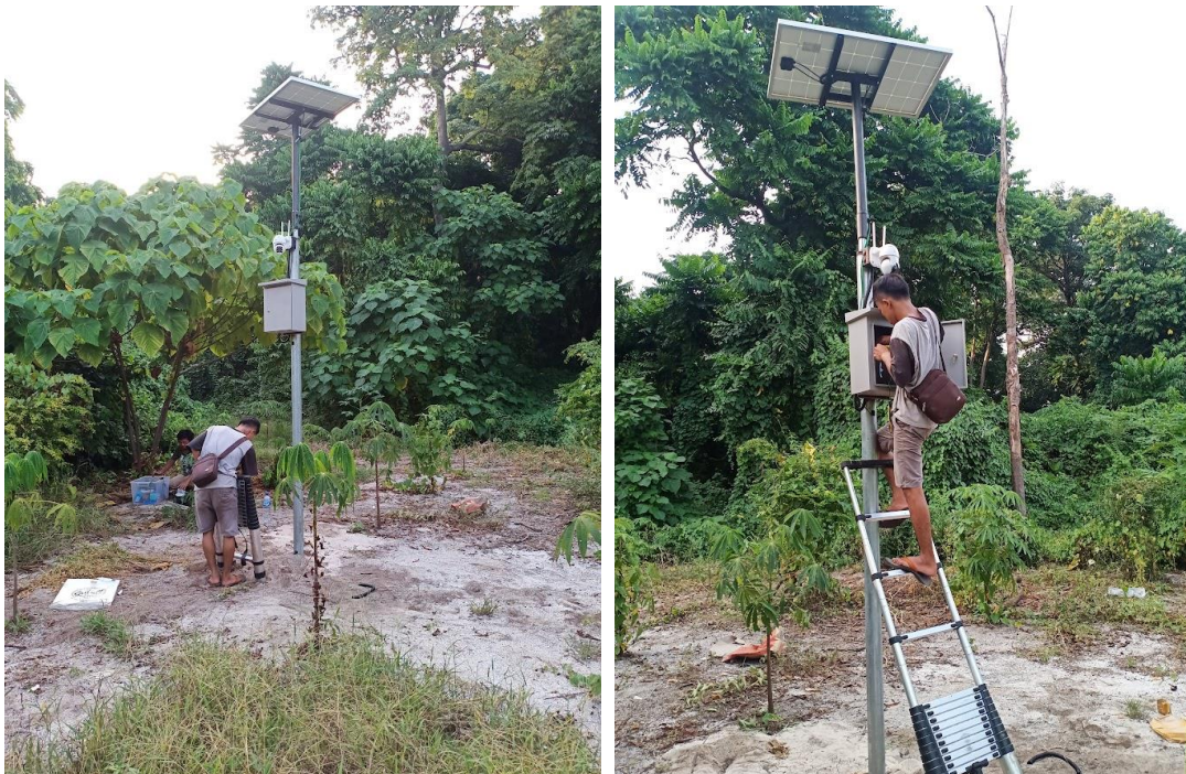
b. Proses pemasangan Solar Panel CCTV Renewable Energy
