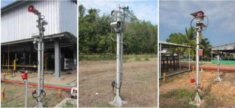
**Gambar.** Fire and gas alarm di PHE Ogan Komering
