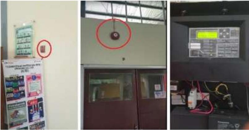
**Gambar.** Alarm dan *smoke detector early warning*
