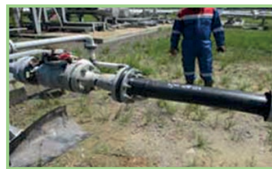
Gambar 10. Inovasi Alat HDPE Pipe Line
