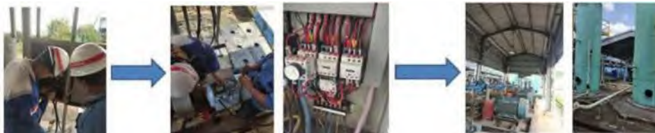
Gambar. Proses gas line grouping
