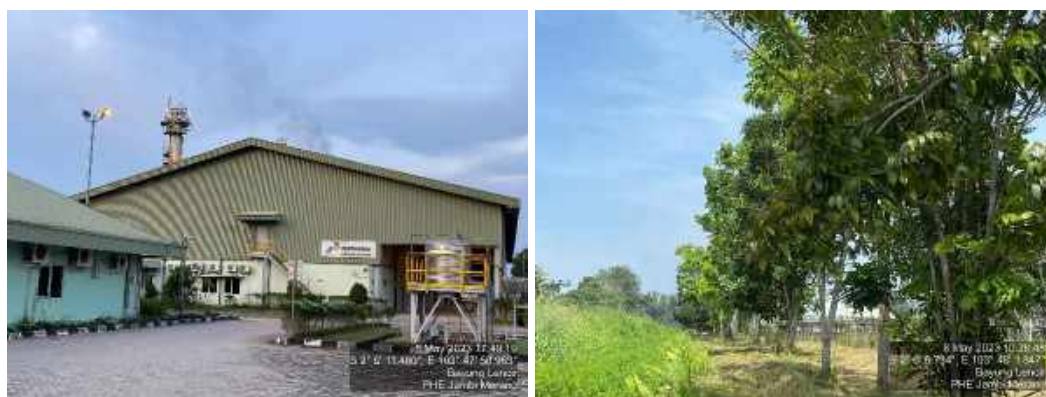
Gambar 3. 8. Area Maintenance Office Work Shop dan CW 7
